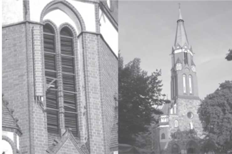
An antenna is camouflaged on the tower of this church in Sopot, Poland. See the close-up on the left. Photo by Piotr Plecke.
