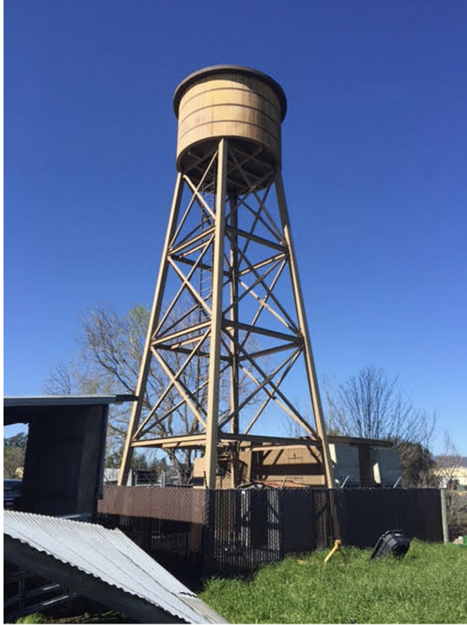
50' fake water tank for concealed cell tower. Regular price $71,700.
