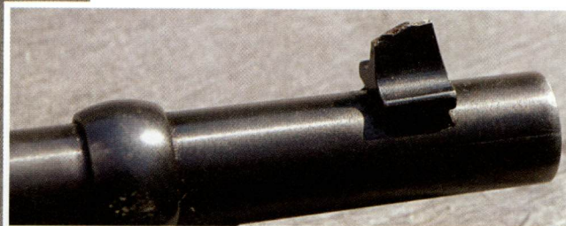
Note the front sight damage.
