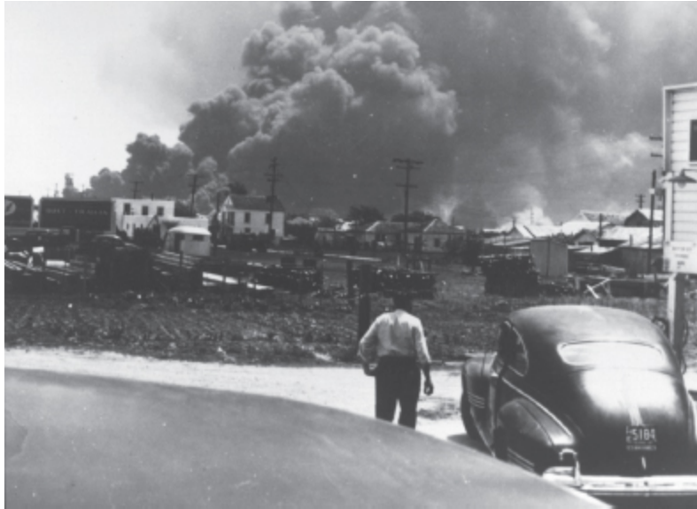
Smoke rising from the destruction at Texas City. (University of Houston)
