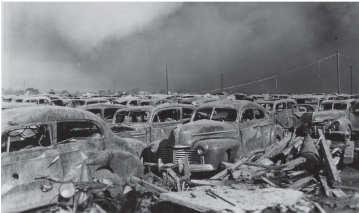
A parking lot a half mile from the Grandcamp shows the power of the explosion's shock wave, which even at that range could cave in the side of an automobile. (University of Houston)
